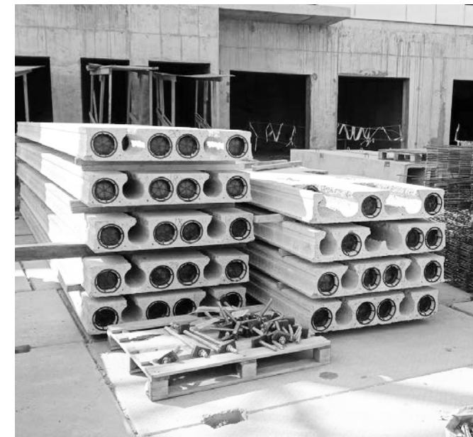
14 RC PRECAST HOLLOW CORE SLABS
