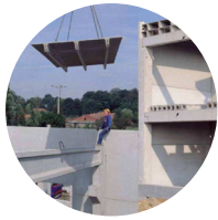
Prefab concrete for the structure
