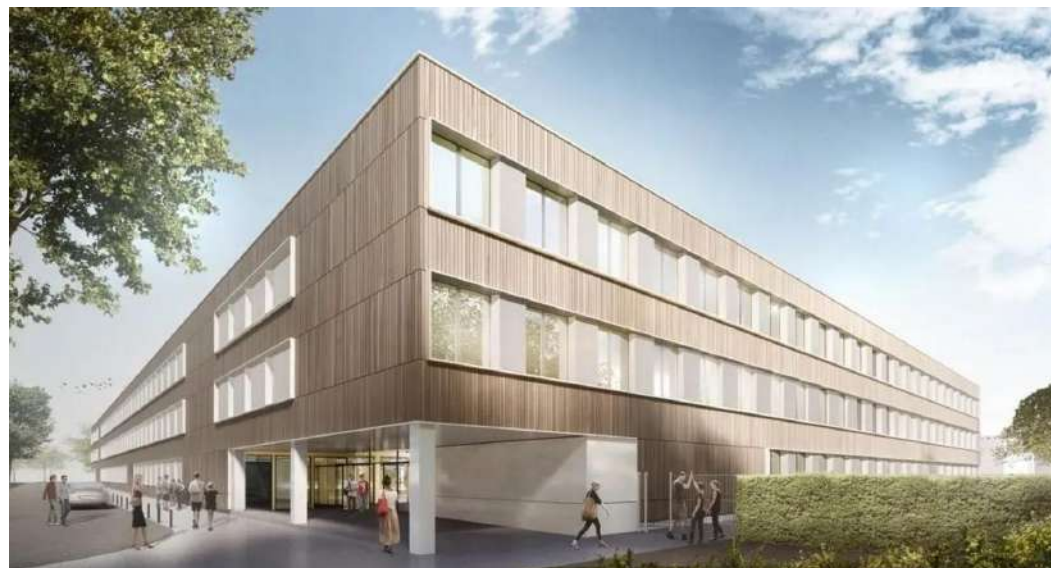
Modular School Built of Wood by gmp · von Gerkan, Marg and Partners Architects Frankfurt, Germany
