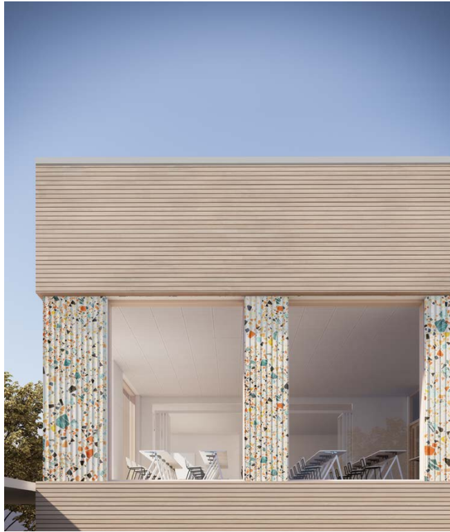
Alternative building facade fragment 2: wood panels and composite panels from recycled materials
